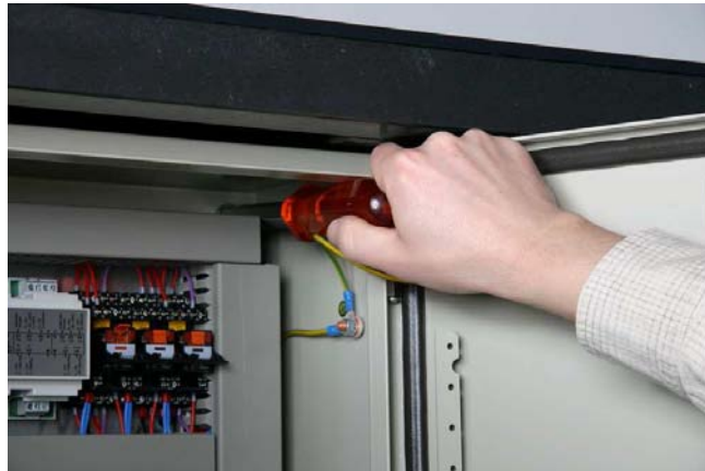
Photo: Loosening the fastening bolts by means of a socket spanner
