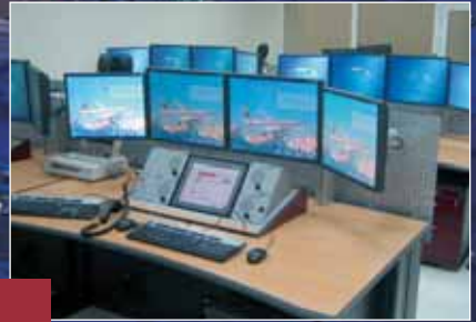
QATAR Qatar Airways, OCC, Doha
