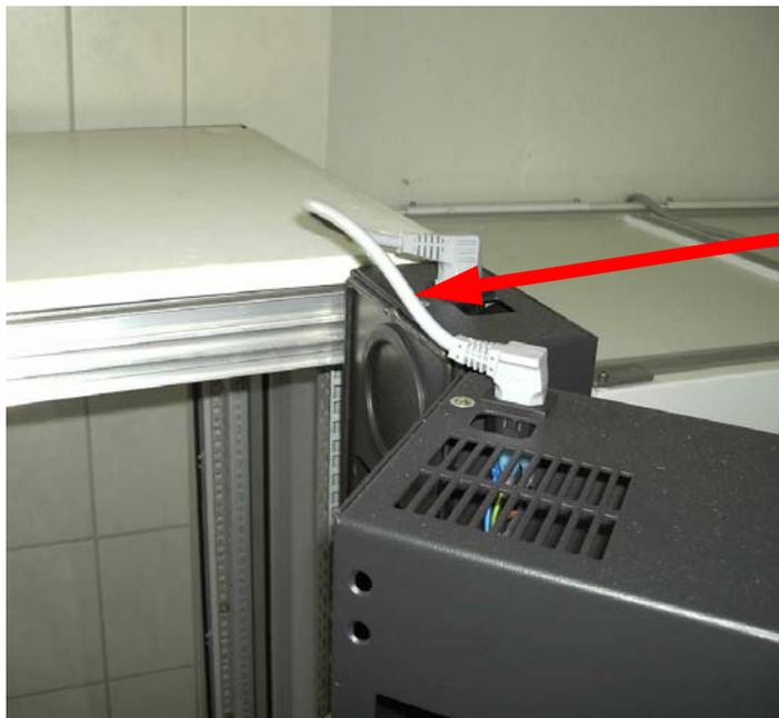
Power link between fan door and heat exchanger
