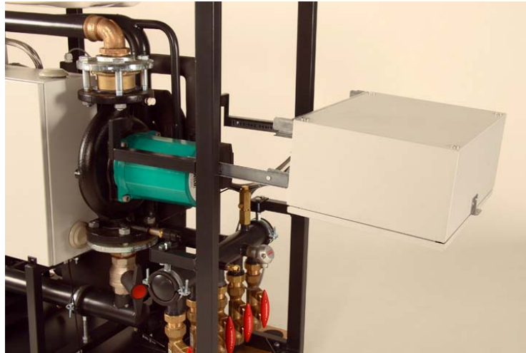
Fig.: pulled and tit out rack
