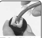
Place the S310 termination cap over the jacket and slide down onto the S310 block.
