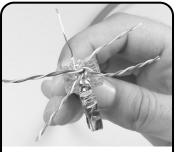
Arrange pairs in an "X". Be sure to follow the wire map on the termination cap label. Push wires one at a time into wire guides.
