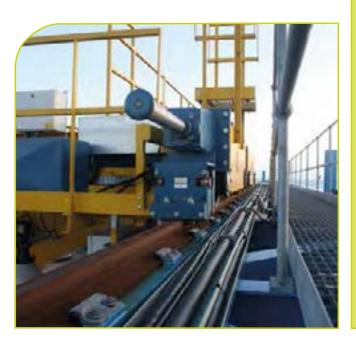
Marshall-Tufflex's corrosion resistant Glass Reinforced Polyester (GRP) cable management trays, which are designed to withstand extreme weather conditions, have been used to carry all power and lighting services to an unloading station at Shoreham Harbour in West Sussex.
