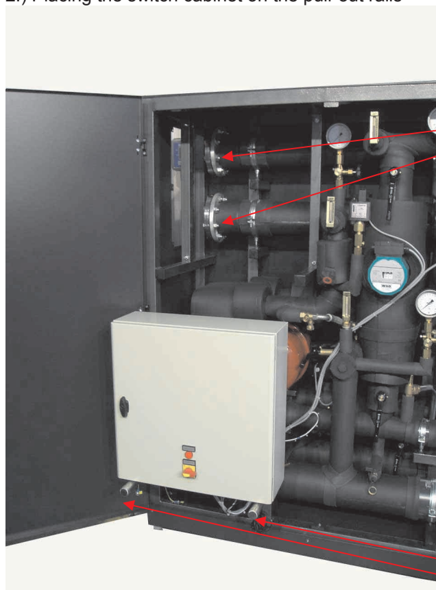
Photo: Switch cabinet, resting on pull-out rails
